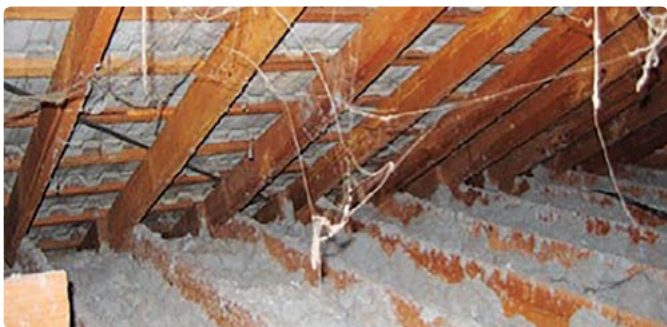
Typical installation of loose-fill asbestos insulation in roof area
